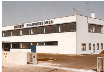
1978: The new BAUER KOMPRESSOREN plant in Drygalski Allee, München
